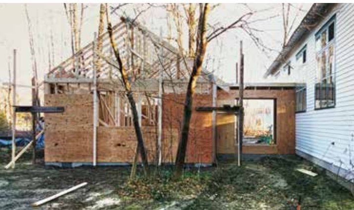
Construction of the annex
